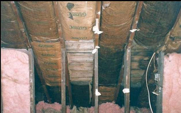
Rotted Insulation
